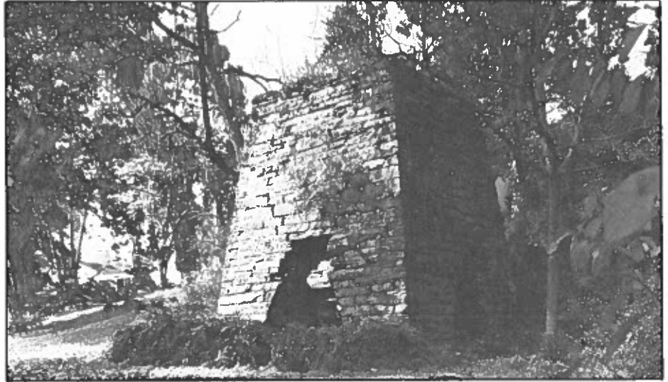
The furnace of the Washington Iron Works erected in 1779 by James Callaway. The furnace cracked around 1850 when the dam broke during a freshet, sending a wall of water on the furnace while in full blast. Note the notch at the top posteriorly for the bridge for filling the furnace with iron ore, charcoal and limestone and the casting floor in front of the furnace where iron pigs, pots, stoves, and so forth were made.
